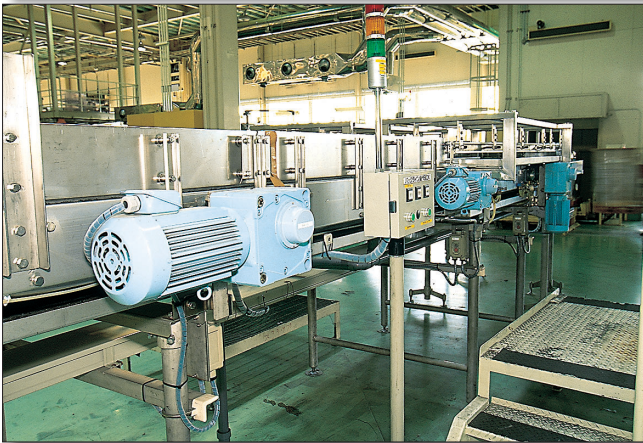
Conveyor lines in breweries
